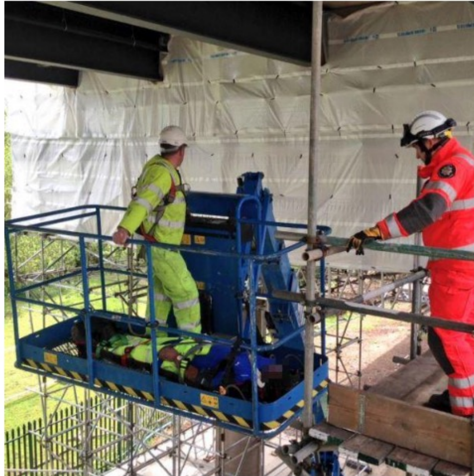
The incapacitated man safely in the platform and ready to go
