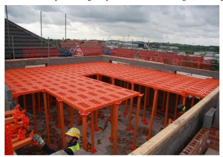
7.1.9 Make sure the corners of the panels are in position on the head plate.
