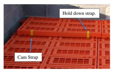
7.1.24 When overlapping panels always put a Leg and Head plate into one of the head plates positions to support the overlapped panel.
