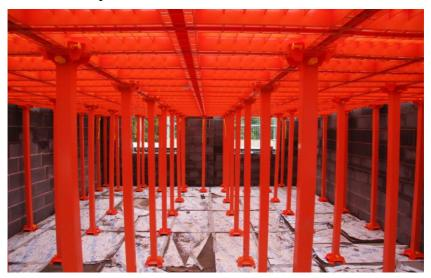
7.1.10 Put the securing pins as you work it saves time later.
