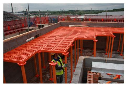
7.1.8 When positioning the panels take care to straighten the legs.
