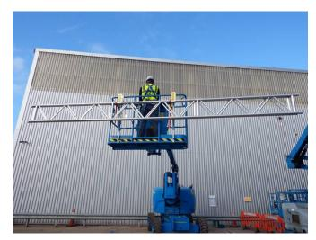
When developing the Safe System of Work, the responsible MEWP Manager and Operator should review the use of materials handling devices available and consider any effect it may have on stability, imposed loads and operational wind speeds of the MEWP. Large materials can act as a sail and the manufacturer may stipulate a reduction in the maximum rated operational wind speed and or reduction of the number of people in the platform.
