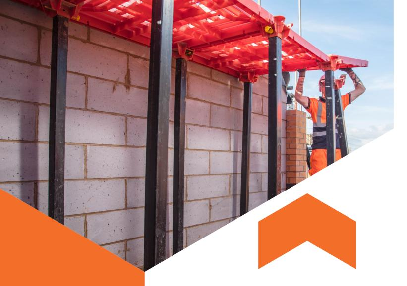
The MacDeck internal fall protection system meets BS EN 12811-1 Part 3 (for structural integrity and safety factor, for use as a general purpose working and safety platform
