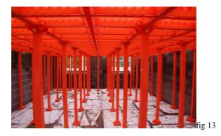
• Put the securing pins as you work it saves time later.
