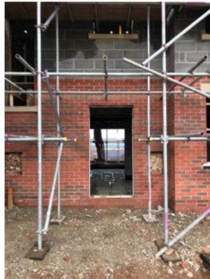
Figure 1. Example of clear access provided through erected scaffolding
