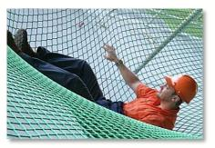
For these reasons, it is not possible to predict the performance of the net should it be subjected to additional loadings in the future. BS EN 1263-1 stipulates that nets should be checked by a competent person after loading. This is generally considered to be the manufacturer (not the installing company) and due to the logistics of this, FASET recommends that safety nets should only be loaded once.
