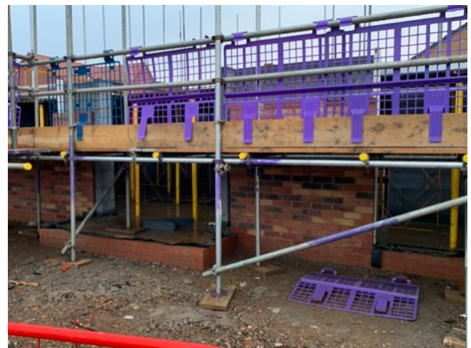
Figure 2. Example of compromised access due to 1st lift scaffold being erected prior to Access Platform Decking system installation
