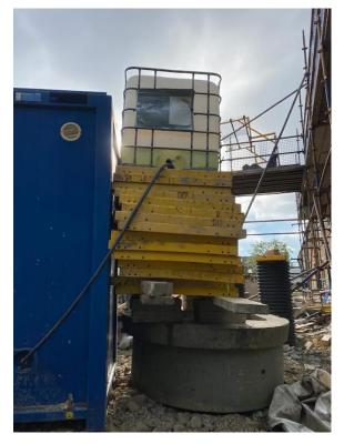
Misusing Access Platform Decking system panels for plant access can cause undetected damage which results in failure when next used correctly.
