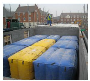
PAS 59: 2014 - Specification for collective fall arrest soft landing systems - is the standard for this type of system. Guidance from the manufacturer for planning and use of Soft Landing Systems should always be considered prior to use.
