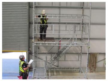
not make that a scaffold". On this basis, just because stair towers use tube and fitting scaffold components does not make them a scaffold either.
