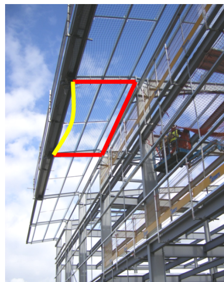
Figure 1. Typical application requiring an eaves bag
