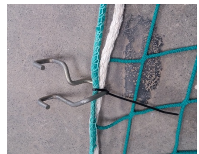
Figure 3. Example of a safety net attachment device secured using a cable tie
