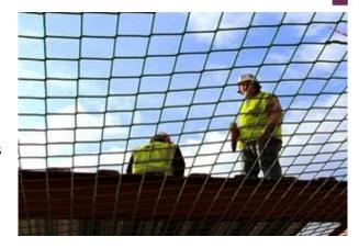
The number of workers protected by an individual Safety Net that complies with BS EN 1263-1 & 2, must be contained within the capacity of the net. Therefore, for a 2m maximum fall height, and allowing 100kg per worker including tools, this would set the recommended maximum number of 2 workers over any section of Safety Net.
