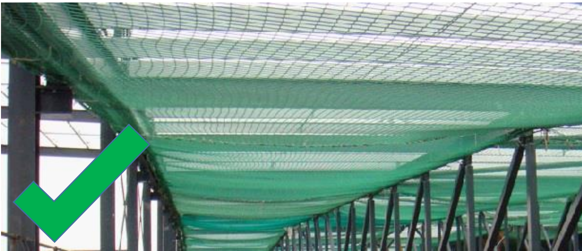
Figure 1. Safety Nets installed with gaps reduced to a minimum
