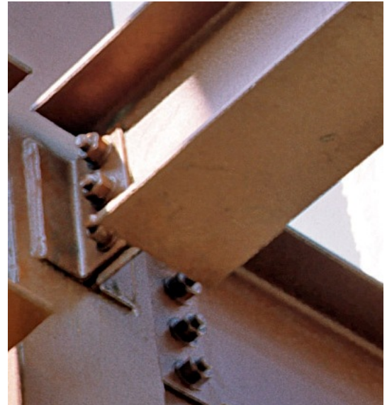
Figure 4. Example of open end in steelwork.
