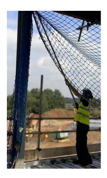
Dependent on the steelwork arrangement, weather conditions and net size, additional fixings such as rope ties are sometimes required at the corners of the net to prevent movement during rigging. Installation of rope ties or similar will involve the rigger working at height to attach them, usually from a footed ladder due to the short period of time required to attach the net, however for longer periods of work, suitable control measures should be considered based upon the degree of risk.
